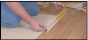
Always start in the middle of a straight run as it is easier to produce a clean join on a straight section as opposed to a curve or corner. Peel backing off the adhesive tape.
