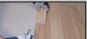
For longer runs try a piece of 3" x 2" to help attach large sections of the binding. Use a glue gun pad when the gun is not in use to avoid glue dripping onto either the floor or carpet.
