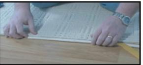
Be sure to run the rope edging parallel to the carpet edge leaving a gap to accommodate the glue gun nozzle.
