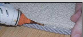
When you are happy with the join and the corners etc. Use the hot glue gun to apply a bead of glue between the binding and the carpet backing, pinching together as you go. Be careful not to get glue on the carpet.
